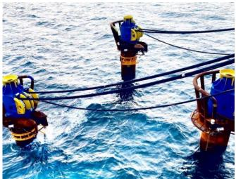
(2) With up to three simultaneously operating drilling rigs, piles were safely and efficiently anchored in difficult soil conditions. © BAUER Group
