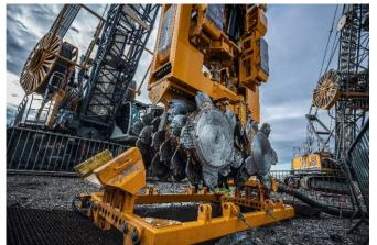
(2) Among other equipment, a BAUER MC 96 duty-cycle crane with BC 48 trench cutter was used for this challenging work.
