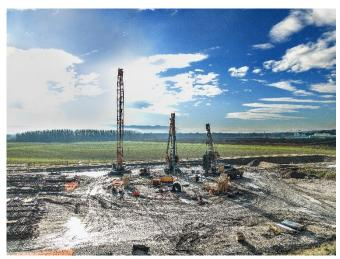
(1) Over an impressive area of 6,500  $m^2$ , the experts from Bauer Spezialtiefbau constructed a shaft 32 m wide and 65 m deep.
