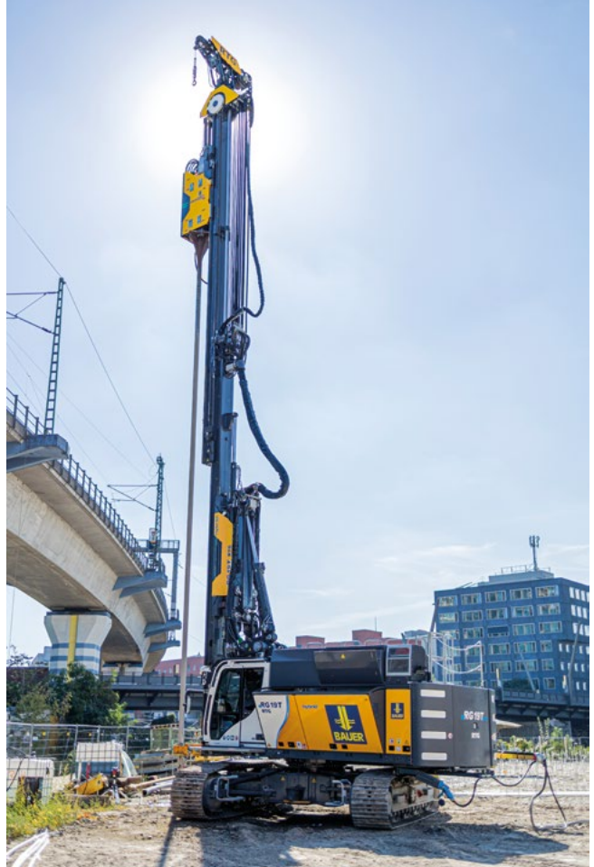
Successful first operation of the eRG 19 T hybrid on a project at Friedrich-Krause-Ufer in Berlin.
