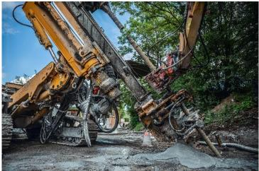
(2) To safeguard the lock, Bauer carries out the necessary injection work with the specially configured KLEMM KR 806-2DB.
