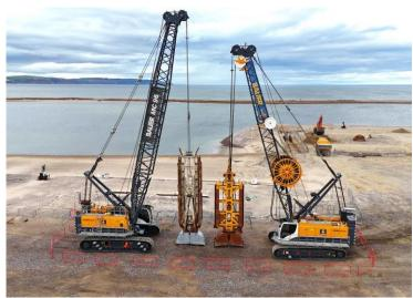
(1) Revitalizing the port in Ardersier, Scotland: Bauer installs diaphragm walls for the front quay wall and rear anchor walls up to impressive depths. © BAUER Group
