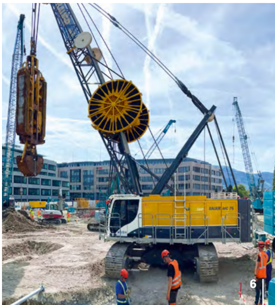
4 | Hungary In the heart of Budapest, the Zugló City Centre is taking shape. Bauer carried out the necessary cut-off wall, anchor and pile drilling work for a office and residential building.
