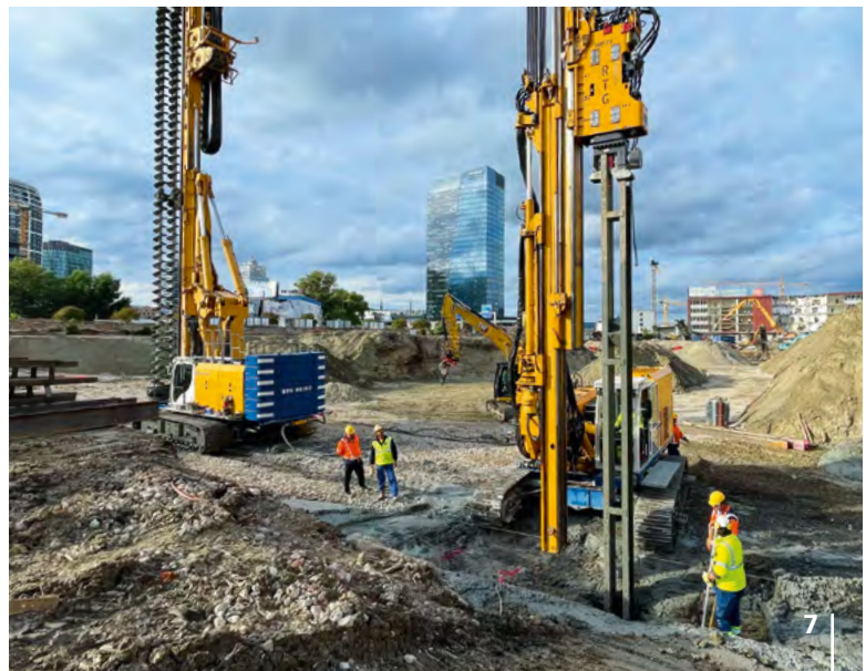
6 | Switzerland In Geneva, Bauer assisted with the specialist foundation engineering work for the new head office of a private bank. Apart from barrette foundations up to a depth of 75 m, diaphragm wall sections were also installed for a 18 m deep excavation pit.
