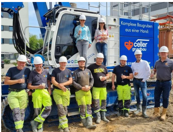
(2) Equipment handover and christening of the new BG 23 H with the name “Julia”
