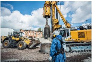
(3) The soil replacement is carried out using large-scale drilling. Special protective suits and an exhaust air purification plant ensure the safety of employees and environment.
