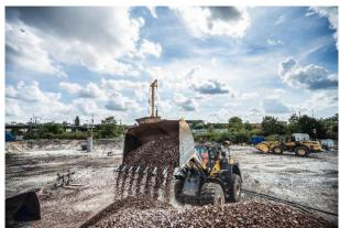
(2) A total of approximately 5,600 m<sup>3</sup> of soil are being excavated and 3,350 m<sup>3</sup> of contaminated material are being replaced to a depth of 9 m.
