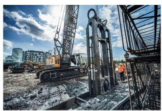
(3) Among other equipment, an MC 64 duty-cycle crane with grab unit is being used for this work.
