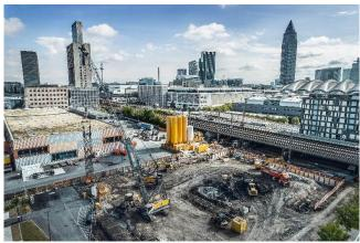
(1) For a new office and hotel high-rise at the South entrance of the exhibition grounds, Bauer Spezialtiefbau is constructing a four-story underground garage and a two-phase diaphragm wall.
