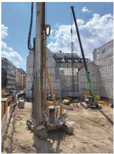
(1) For the retaining structure, Bauer is constructing a total of 298 piles using the double-head drilling system.
