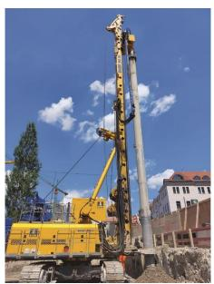
(2) With a BG 30, piles are drilled up to a depth of 18 m.
