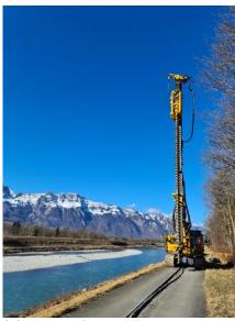
(2) As a safeguarding measure, a 530 m long and 10 m deep cut-off wall was constructed using the mixed-in-place method.
