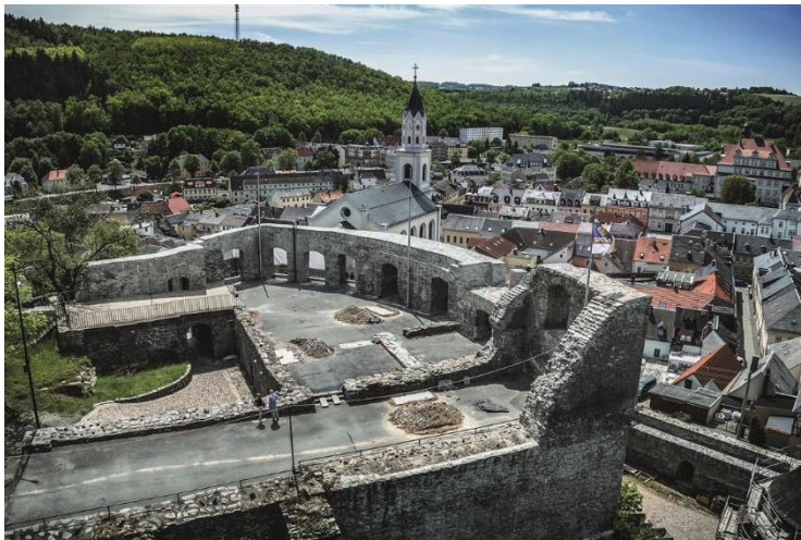
(1) The rehabilitation work is planned to conclude this summer.
