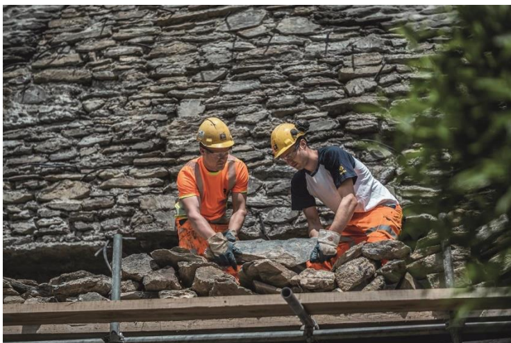
(4) In order to fulfil the requirements of a protected monument site, the historical appearance of the natural stone walls needs to be restored as closely as possible.
