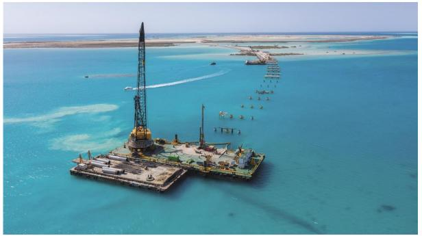
Multiple bridges are being constructed for a new, sustainable recreation area by the Red Sea. In addition to three test piles, Bauer constructed a total of 124 piles for this project. © BAUER Group
