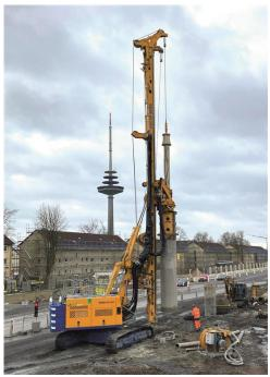
Bauer is constructing a total of approximately 20,000 m<sup>2</sup> of secant pile wall. © BAUER Group
