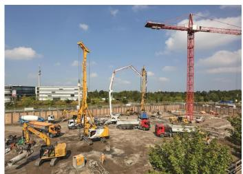
(1) A total of 301 piles with a diameter of 880 mm and a length of up to 24 m were installed.
