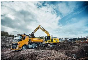
(3) A 30-ton excavator is used to excavate about 26,000 m³ of contaminated soil.
