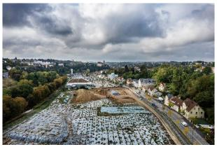
(1) The Bauer Umwelt Division of BAUER Resources GmbH is carrying out soil remediation work on the site of a former tannery and is preparing the excavation pit for the construction of a new nursing home.
