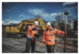
(2) The area was surveyed with centimeter precision using a drone and rover rod.
