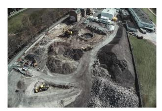
(3) A total of 9,100 m<sup>3</sup> of material was excavated and disposed of.
