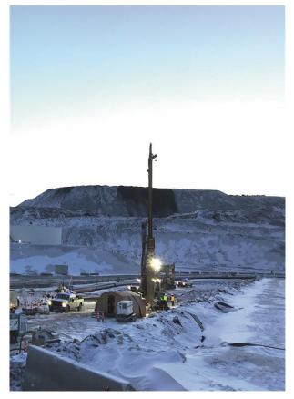
(1) Around 170 km north of the Arctic Circle, BAUER Foundation Corp. carried out field tests using the jet grouting and Cutter Soil Mixing methods.
