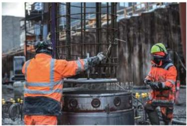
(2) The installation of the BAUER lift cells was carried out during the day, while injection work was carried out during the night shift to ensure completely vibrationless working conditions.
