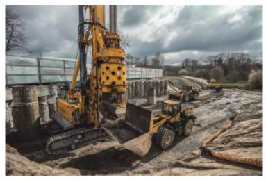
(2) A total of approx. 3,500 m³ of soil must be excavated and 6,000 m³ of contaminated soil material will be replaced to a depth of 15 m using large-scale boreholes.
