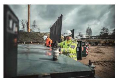
(3) Contaminated material is removed and disposed of in gas-tight containers.
