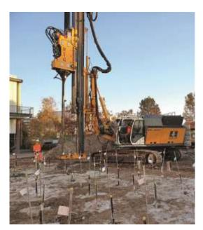
(1) In order to seal the excavation base from the Quaternary aquifer sands, a low lying BAUER LWS silicate gel base was realized.
