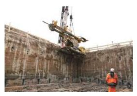
(2) The grouted anchors, with four to six strands and a length of approx. 17 m, were created using the rotary percussive drilling method.
