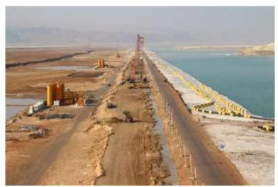
In just 16 months, BAUER International FZE constructed around 112,000 m² of cutoff wall over a length of 4.2 km for the rehabilitation of a dike at the Dead Sea. © BAUER Group
