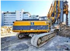
(2) The mixed-in-place method (MIP) developed by Bauer has proven to be a particularly suitable specialist foundation engineering method for the project. © Guido Anacker
